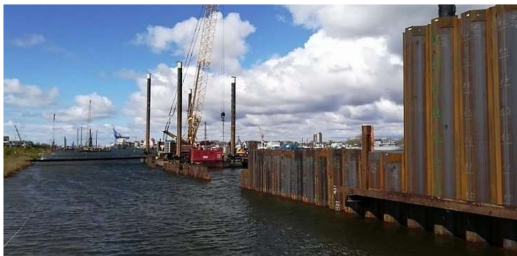
3.3.9 Fig. Example of the installation of a driven retaining wall near the Smeltė Botanical Reserve (progress of works – the wall is almost fully driven at the very front, closer to the camera – still
